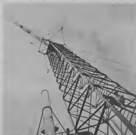
THE BRAZILIAN Miguel Pizanelli climbed several times to the top of this second highest structure in the refinery (307 feet). E BRAZILERO Miguel Pizanelli a subi varios bez na top di e segundo estructura mas haltu den refinaria (307 pia).
